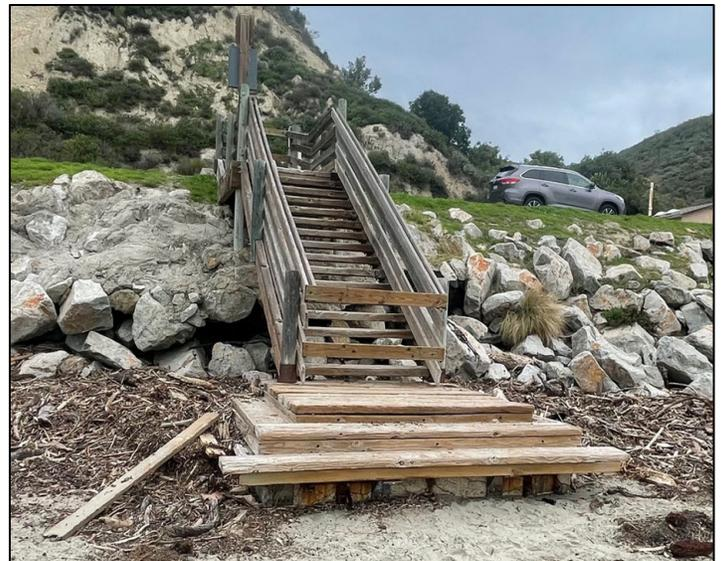
**Figure 2. Damaged wooden base to stairs**
