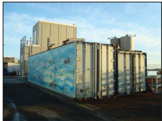
MBCFO Cold Storage Facilities
