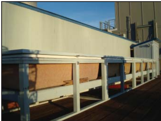
Live Fish Holding Tanks, MBCFO Wharf
