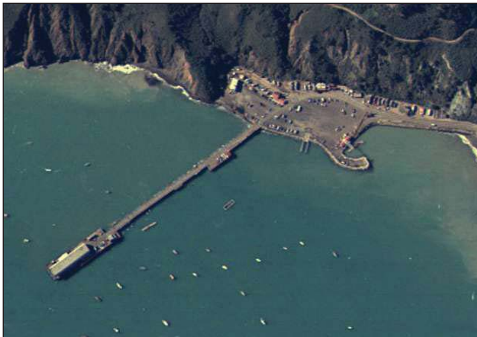
FIGURE 5.2 HARFORD PIER, PORT SAN LUIS HARBOR DISTRICT
