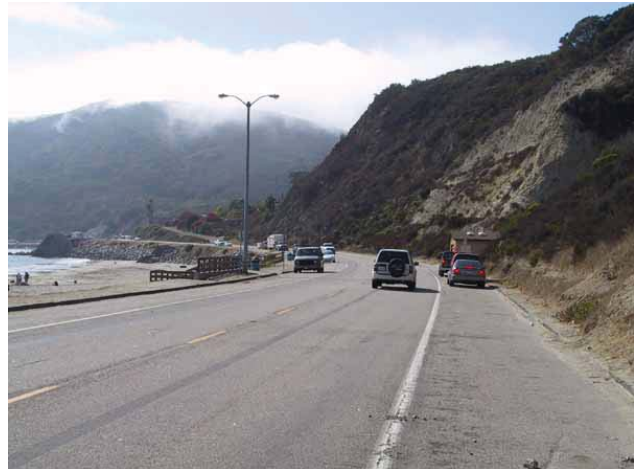
Avila Beach Drive provides the only vehicular access to the Port. The roadway is shared by motorists, bicyclists and pedestrians.
